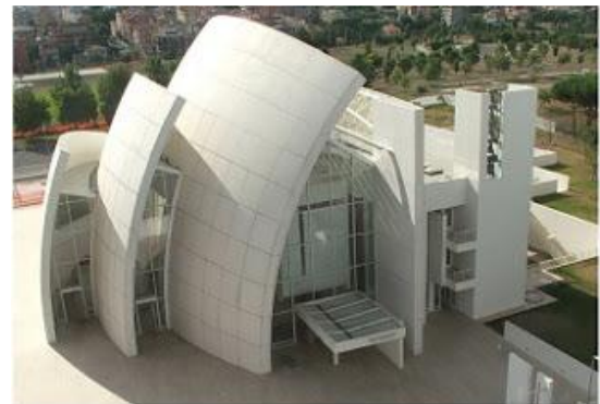
Fig.3. Building made by using self-cleaning concrete (Church “Dives in Misericordia”, Rome, Italy)
